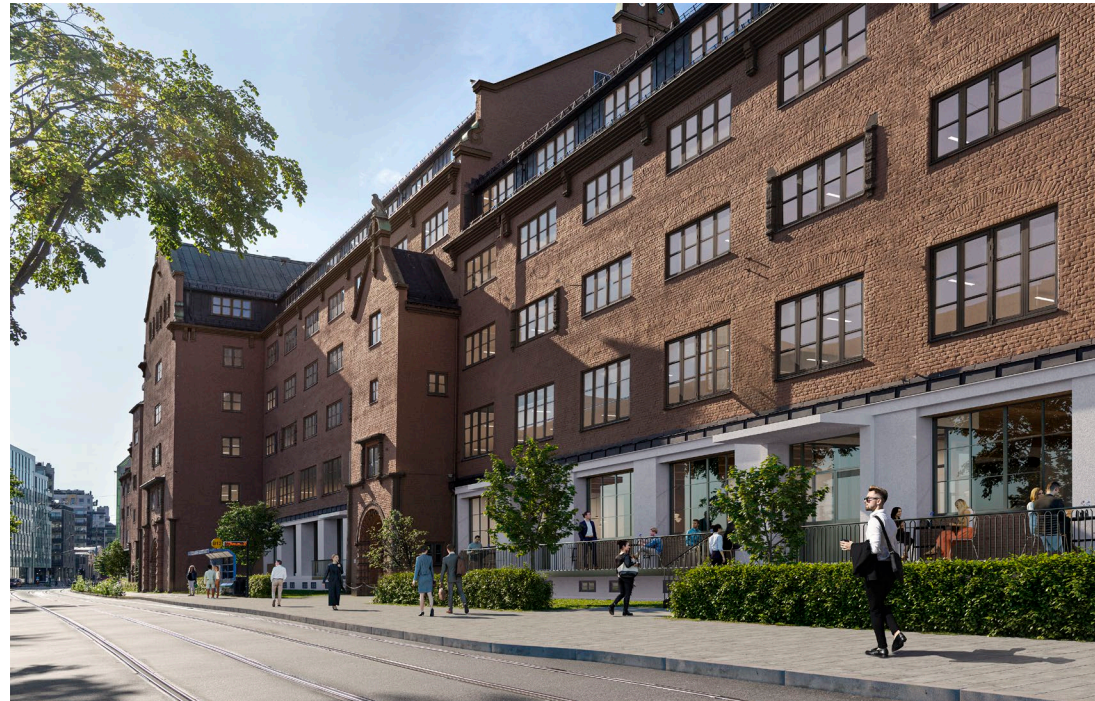
Schweigaards gate 15 in Oslo
