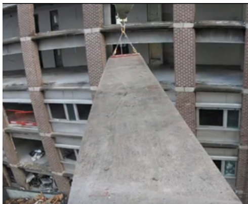
Hoisting the hollow core slabs out of R4. Video clip from NRK
