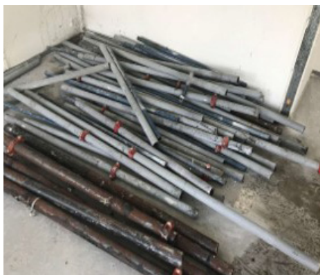
Used sprinkler pipes, dismantled from U2. Photo: Christoffer Siopan Engtrø
