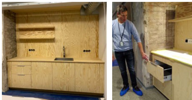
Fully installed cabinets with new fronts made of 15mm plywood. Photo: Lars Ulrich Nielson/LUN and Anne S Nordby
