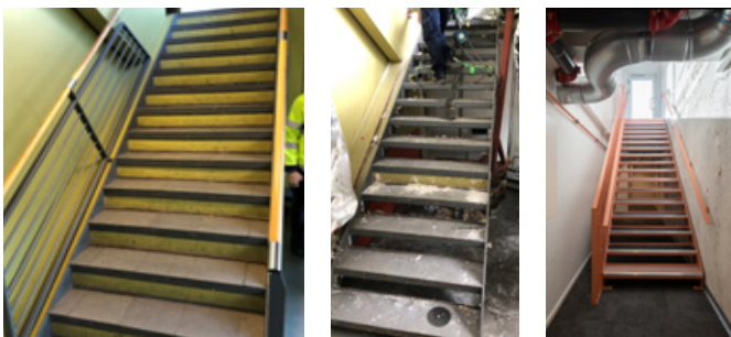
1–2: Stairs before and during dismantling from St. Olavs Plass 5. Photo: Rune Andersen
