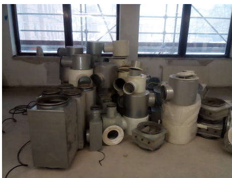
Used, round ventilation ducts and duct elbows – dismantled and roughly sorted in KA13. Photo: Anne S Nordby
