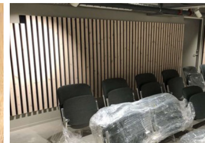
Completed booths and cladding made of used slats on the back wall of the cinema room. Photo: Rune Andersen
