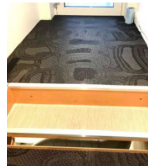
Bolon flooring (vinyl) installed on the stairs. Photo: Annette Thorsrud
