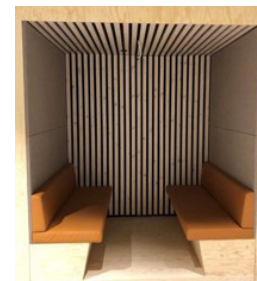
Completed booths and cladding made of used slats on the back wall of the cinema room. Photo: Rune Andersen
