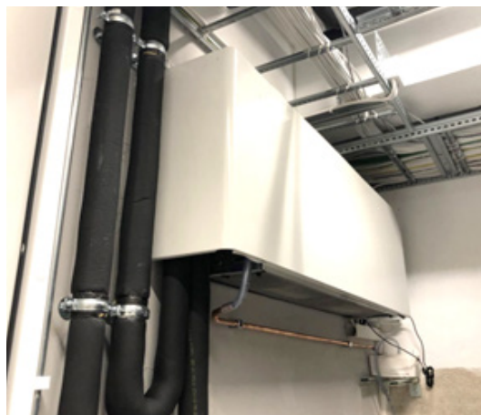
The reused fan coil unit installed in the computer room in the basement. Photo: Rune Andersen
