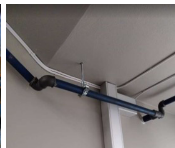
Used sprinkler pipes, completed installation. Photo: Anne S Nordby
