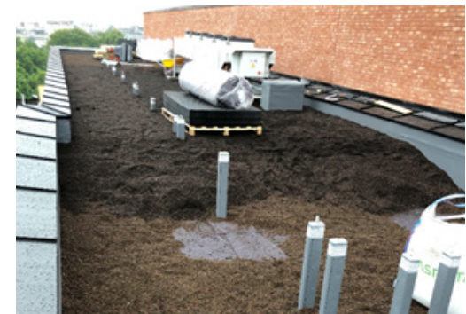
Recycled soil placed on the roof. Photo: Rune Andersen
