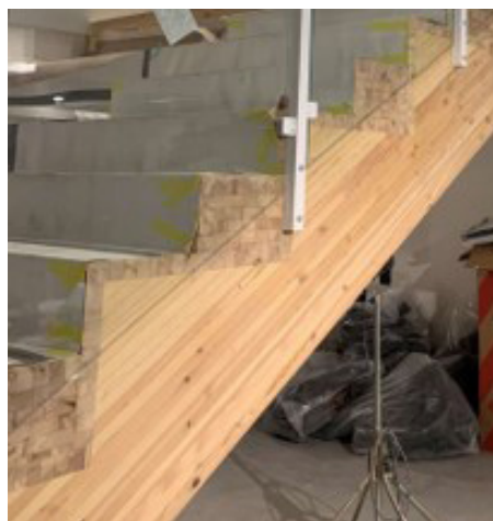
Side wall with visible end wood. Photo: Randi Lunke
