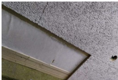
The mineral wool ceiling panels were used for sound absorption on top of the fixed wood wool cement panels. Photo: Anne S Nordby
