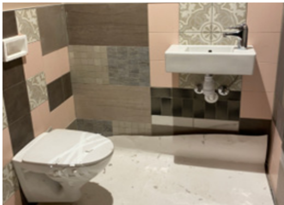
1-2: Selection of surplus tiles and test laying. Photo: Kristine Aassved Storeide
