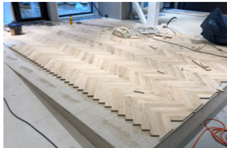
The parquet slats during installation.
