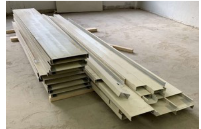
Cableways after dismantling. Photo: Randi Lunke
