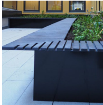
The seat panels made of recycled plastic are mounted onto the steel panels. Photo: Janicke Ramfjord Egeberg
